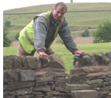
Lengthsman, Dave Bridge, puts the finishing touches to the new stile.
