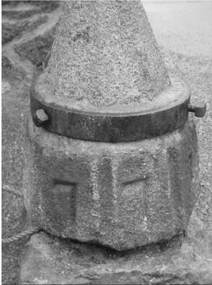
The capping stone was removed during renovation in 2000 and re-bedded. The limestone base is visible. The iron collar was removed.
