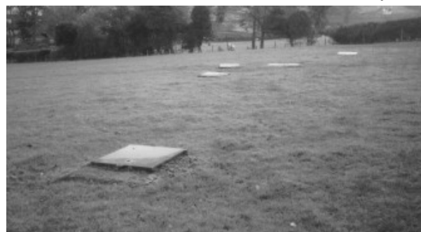
Inspection covers to the reservoirs on Denbury Down
