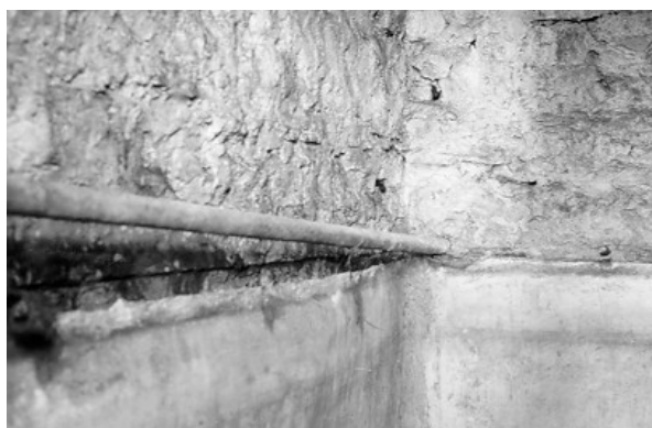
The tank inside with redundant pipe to outside
